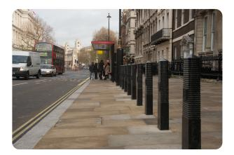
Bollards | Static Manufacturer:ATG Access Standard Tested To: PAS 68:2005 Performance rating: V/7500[N2]/48/45:0/0.0
