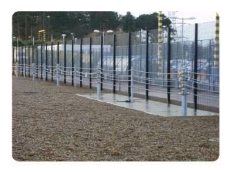
Perimeter Barriers | Vehicle Manufacturer:Safetyflex Barriers Standard Tested To: IWA 14-1:2013 Performance rating: V/7200[N3C]/80/90:13.7
