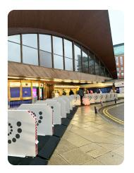
Perimeter Barriers | Modular Manufacturer:Marshalls Standard Tested To: IWA 14-1:2013 Performance rating: V/2500[N1G]/48/90:5.2
