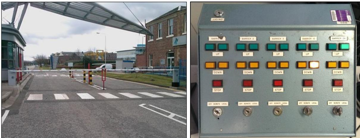
Figure 1: A typical VACP including active VSBs (left); control panel for an active VSB (right).
