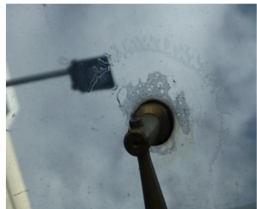
Figure 4: Delamination around a point fixing
