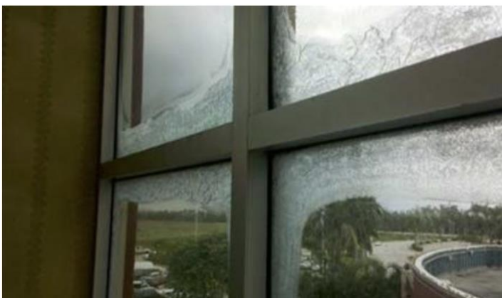
Figure 3: Edge delamination in framed glass
