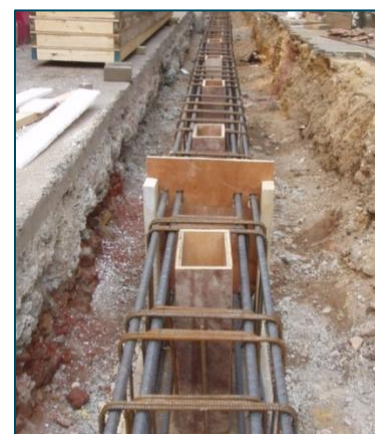
Figure 1: Deep Foundation (illustration and photograph)
