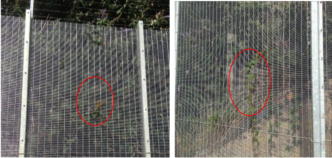
Figure 144a & b: Vegetation growing through fences (circled) triggering false alarms on the Perimeter Intruder Detection System (PIDs)
